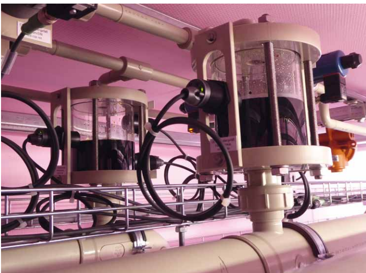
A look at the interior of the JenaBatteries device.
