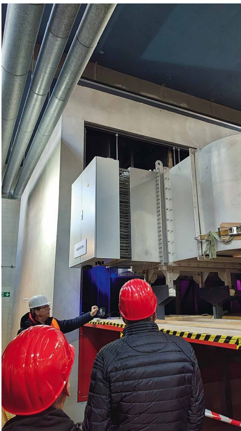
At the opening of the new installation in Berlin last December, Lumenion showcases its 4-ton steel block, which stores at up to 650 degrees Celsius.
